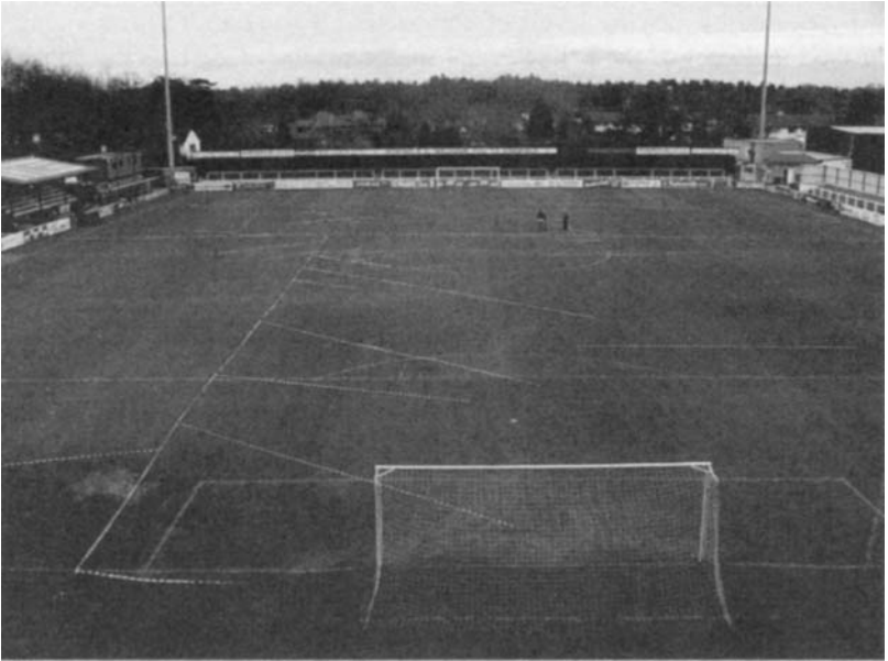
Figure 13.10 Photograph showing the marked-out drainage pattern
