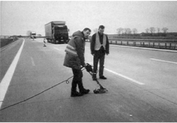
Figure 9.24 Radar measurements with the 1.5 GHz antenna and survey wheel along a false joint
