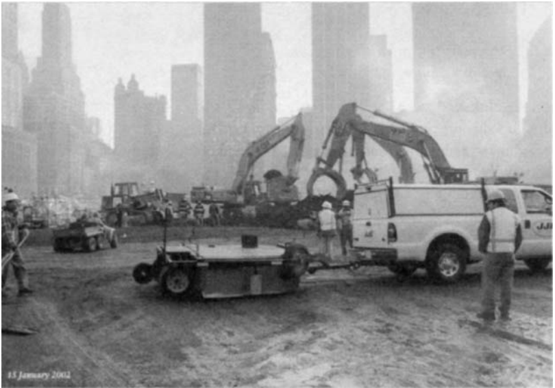
Figure 13.5 Underground radar tomography at ground zero
