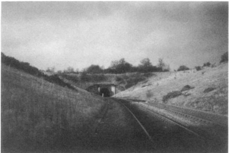
Figure 9.29 Gonerby railway tunnel (courtesy British Rail)
